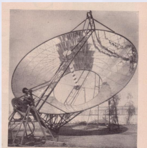
This strange looking machine is a solar engine erected at Pasadena, Calif. The ring of mirrors concentrates sun's energy and the outfit is reported to have produced about four horsepower
