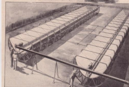
At top, heating water with a solar boiler at the Soviet's experiment station at Tashkent. Above, view of the most successful solar power apparatus thus far made. It was erected near Cairo, Egypt, and uses boilers placed at focus of horizontal reflectors
